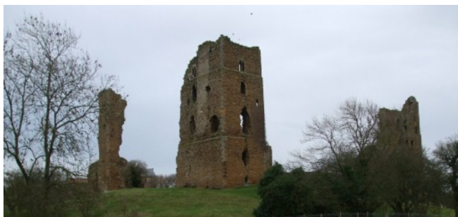
Sheriff Hutton Castle on the route of the Yorkshire Castles Way Photo courtesy of Stephen Down
